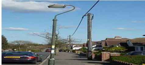
Figure 1: Example of an Insulated Bundle Electric Network
